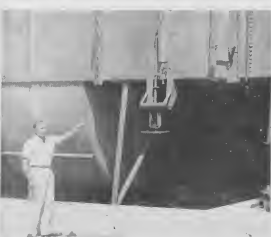
J. Landau, Cracking, earned Fls. 100 by suggesting a better regulating device for stack dampers. Here he points to the control which permits setting the damper in any position and assures against any accidental shut-off.
